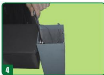
4 Align the screws of lighting fixture with mounting hole of lighting pole and fasten them with stainless steel flat washer, spring washer and nut in place tightly.
