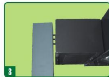
3 Put wire leads of lighting fixture through the wire outlet hole of lighting pole.
