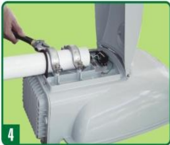
4 Set the level of the fixture and tighten the bolt at the torque of 13~15 N·M.
