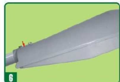
6 Adjust the angle of the fixture and fasten the hex bolt M10×35 with torque at 13~15 N·M. correctly.
